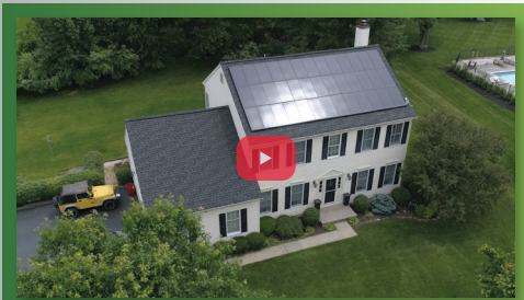
Pegasus Solar Mounting: Composite Shingle Roof Installation
